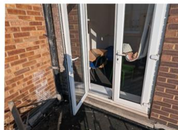
Windows to first floor bedspaces along Tottenham Lane. Windows are placed on restrictors and kept locked for safeguarding purposes
