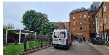
External courtyard / Service yard
